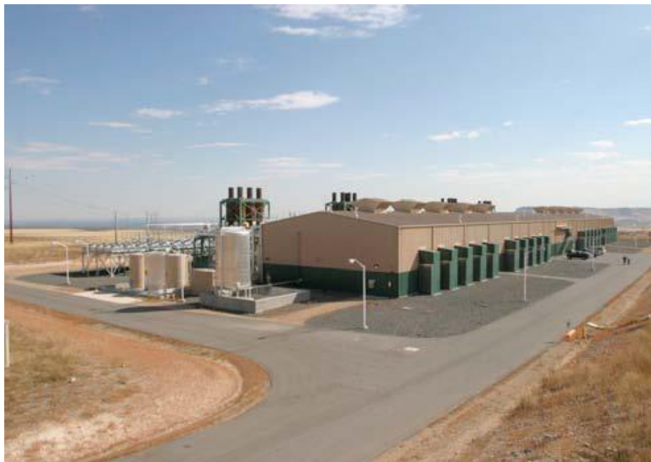
The Plains End I and II grid stability power plants are located in COLORADO, USA and consist of 20 x Wärtsilä 18V34SG engines and 14 x Wärtsilä 20V34SG engines with a total output of 231 MW. The gas fired power plant was delivered in 2002 and 2008.
